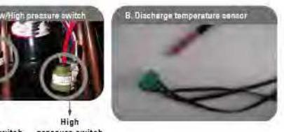
Ensure the compressor operate in the safe range, and prevent damage caused by refrigerant leakage.
